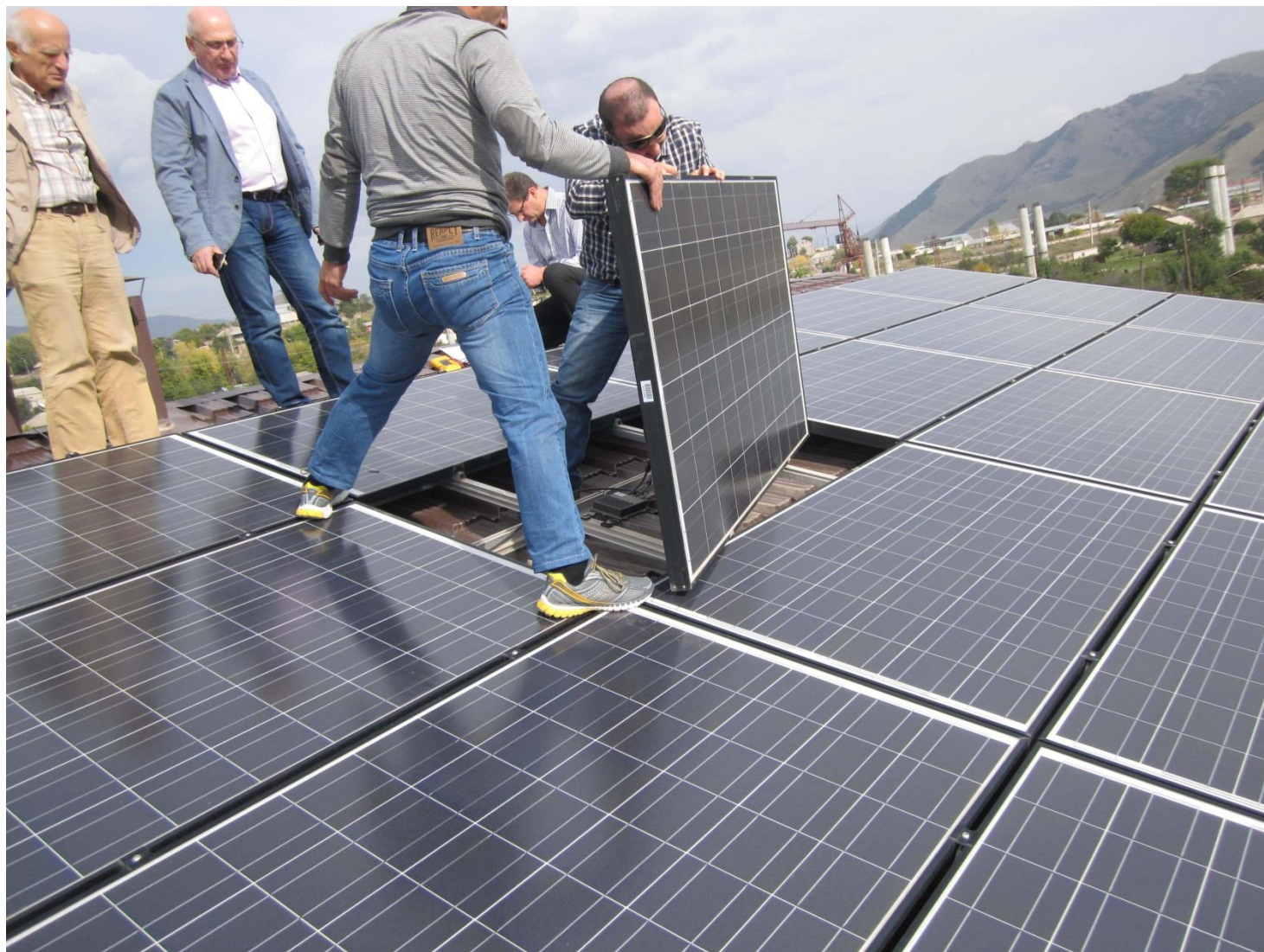
17 KW PV station installed at the roof of YMCA building in Spitak, October 06, 2015
