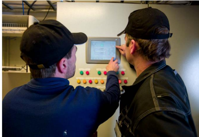
Figure 8: Example of an operational routine at one of the biomass boilers in Norway
