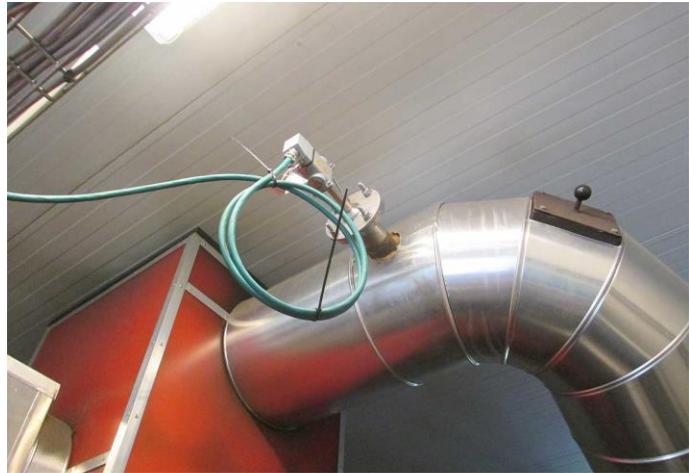
Figur 7: O 2 sensor at the exhaust of a biomass boiler
