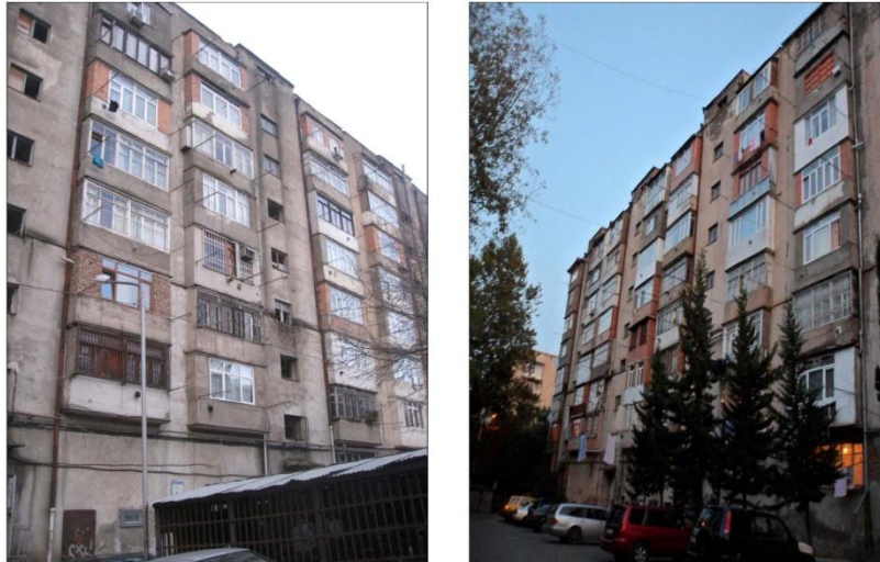
Fig.3. Northern façade of the building
