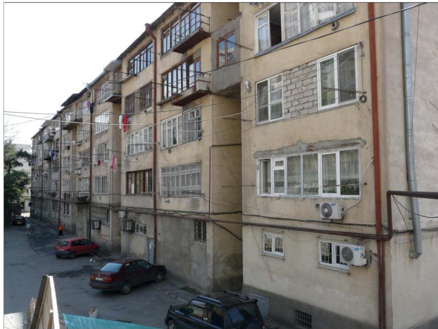
Fig 3. North back facade
