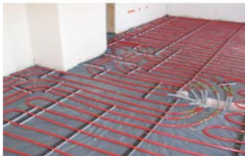
Figure 3.7. In a modern under floor heating system pipes are laid into the floor, usually a solid screed floor. 23
