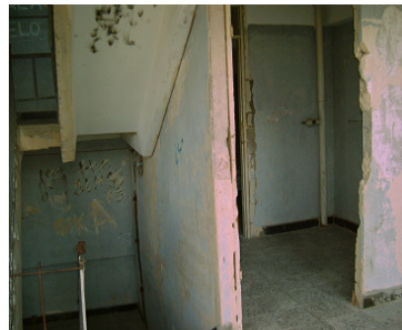
Fig. 2.1.4 stairwell and entrance to corridor in Petrisi str.
