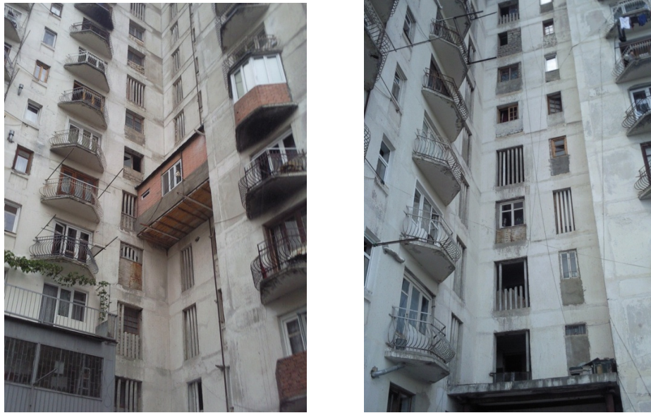
Fig.2.1.5 General view of the building in Vazisubani district
