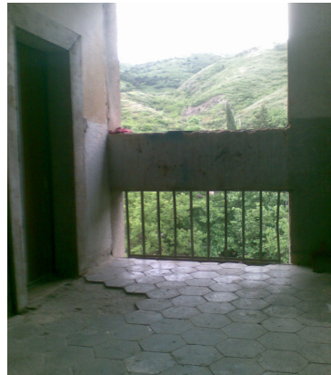
Fig.2.1.2 Stair-well in Gorgasali str.
