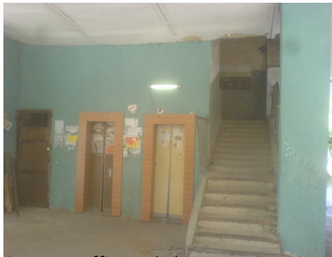
Fig. 2.2.3 Energy efficient lighting in Digomi massive
