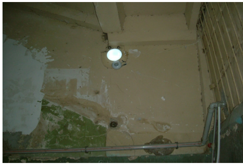
Fig. 2.2.1 Motion sensors in Digomi massive
