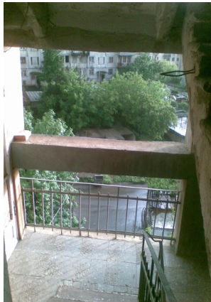
Fig. 2.1.1 Stair-well in Mukhiani
