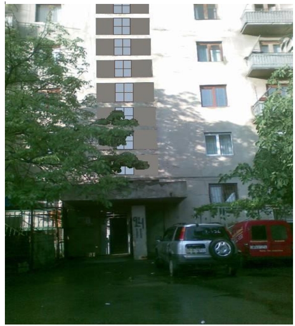
Fig.3.2. Mukhiani. Masonry and new arranged windows
