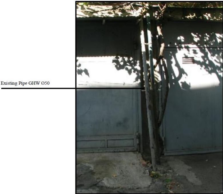
Existing Piping in the Yard
