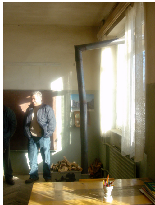
Figure 7. Loose, poorly hung stove pipe.
