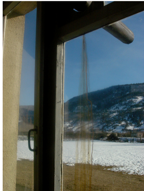
Figure 4. Creosote leaking from a stove pipe onto a window.
