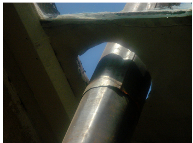
Figure 5. Typical air leaks around stove pipe.
